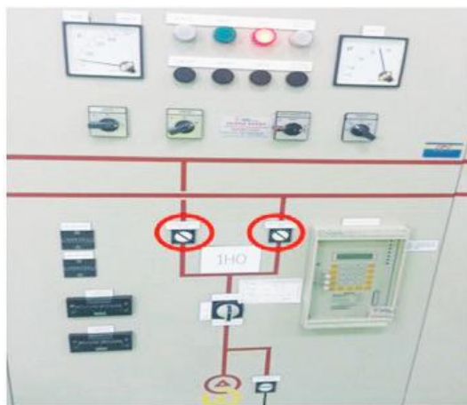
The indicator and indicator lights should be properly installed and should indicate the current status of supply at the switchboard either in the on or off mode.
