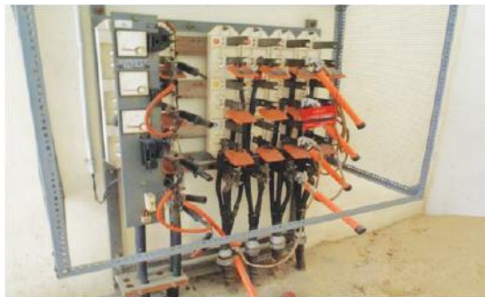
The circuit of the low voltage panel should be earthed properly, exclusive of the consumer distribution circuit for effective earthing.
