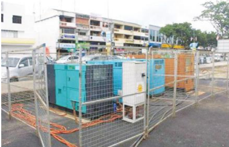
A poorly-managed wiring installations
