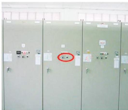
The indicator and indicator lights should be properly installed and should indicate the current status of supply at the switchboard either in the on or off mode.
