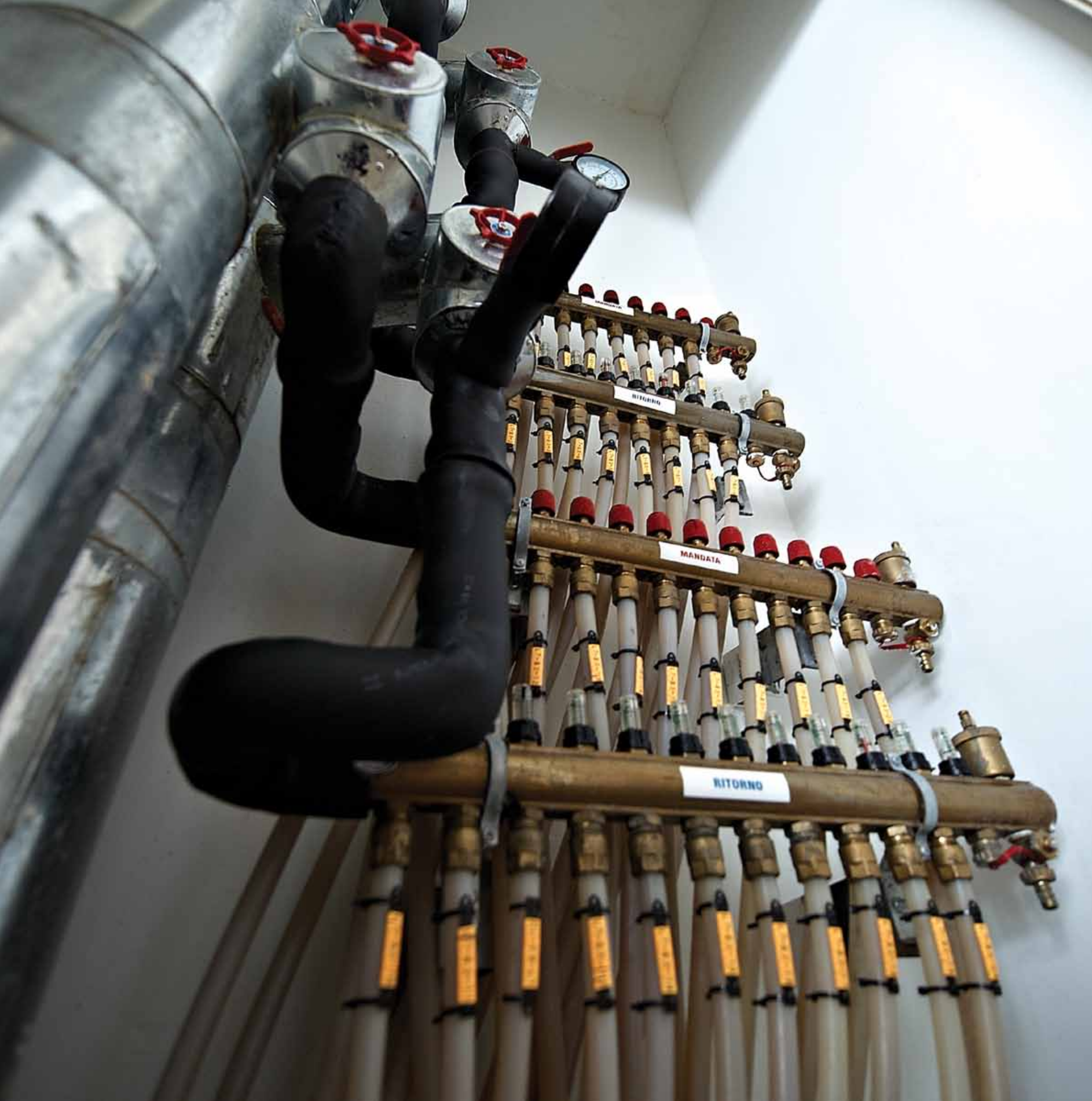
▶ Manifold riser for slab cooling pipes (PERT pipes).
