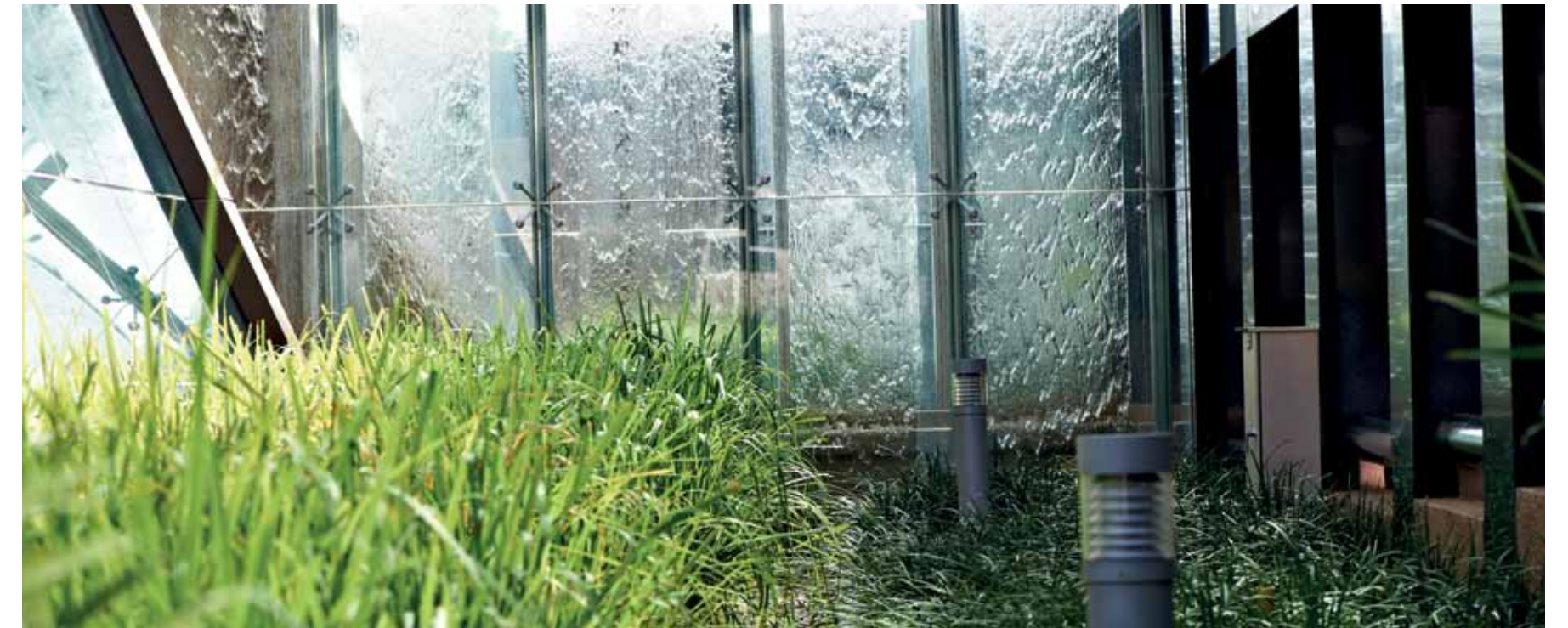
Landscape garden on the ground floor helps reduce heat gain into the building.
