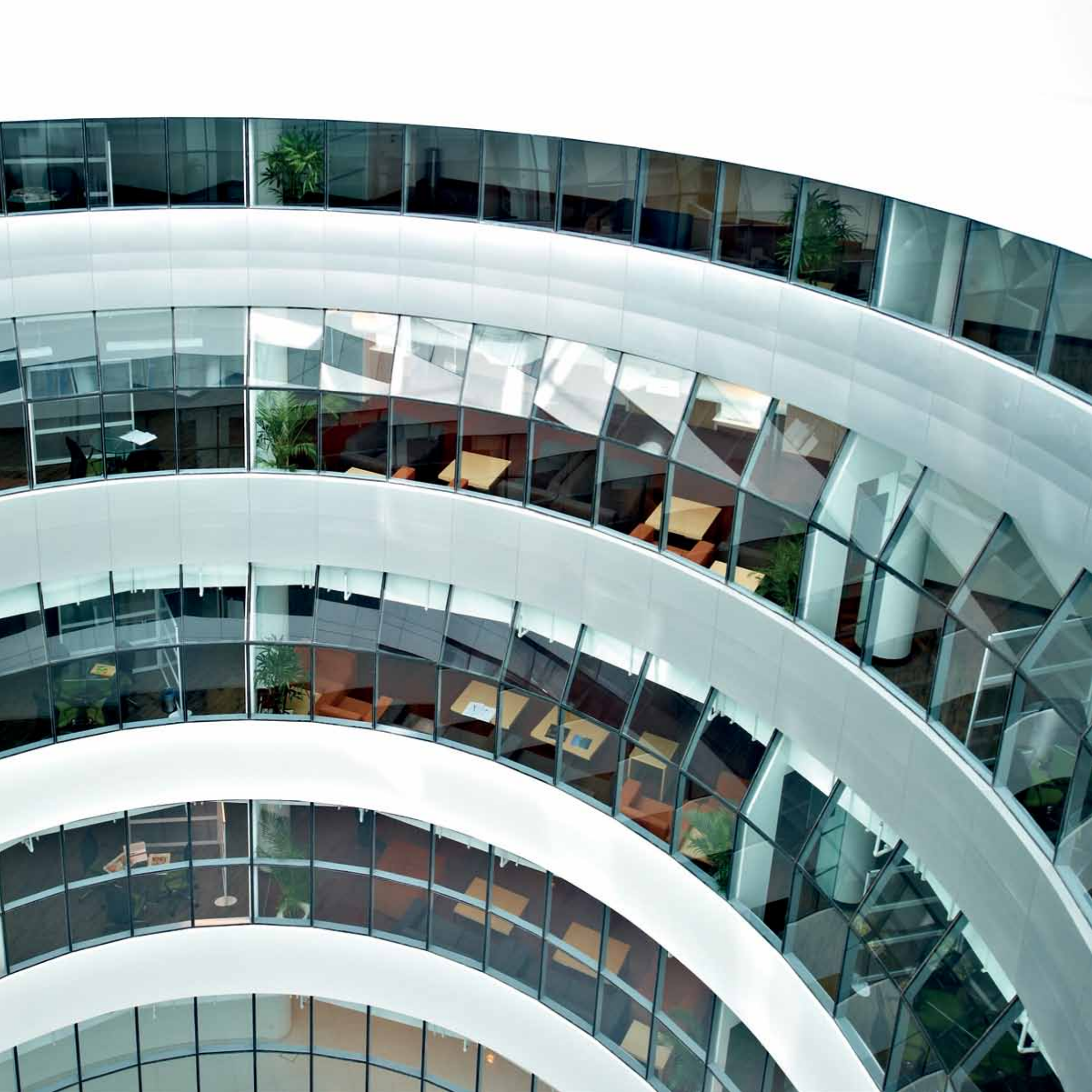
▶ The atrium with Tannenbaum reflective panels on the 4 th and 5 th floor helps to reflect light to the lower floors.
