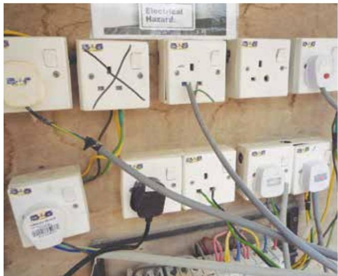
Unsafe wiring in a temporary installation at a construction site
