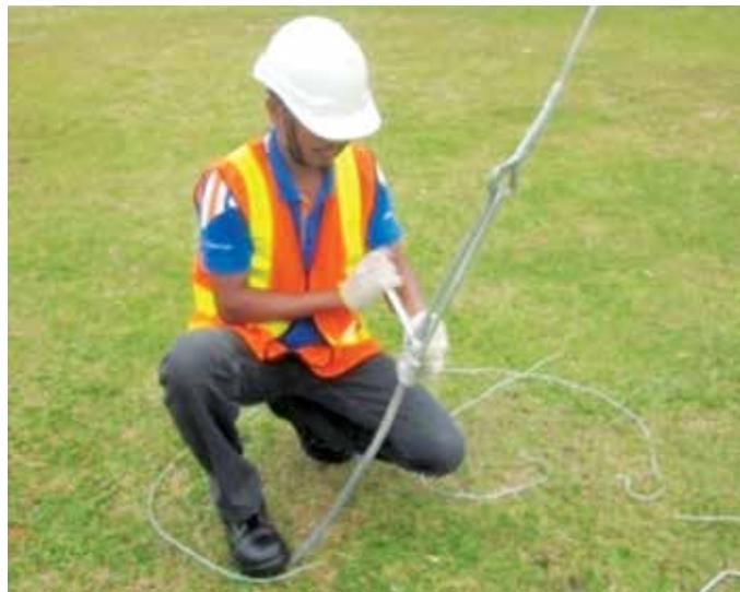
Cable-lacing test for low-voltage overhead line for the A1 maintenance operator category
