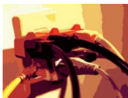
Never connect too many power plugs to a single power outlet as this will increase the risk of overloading and equipment damage.
