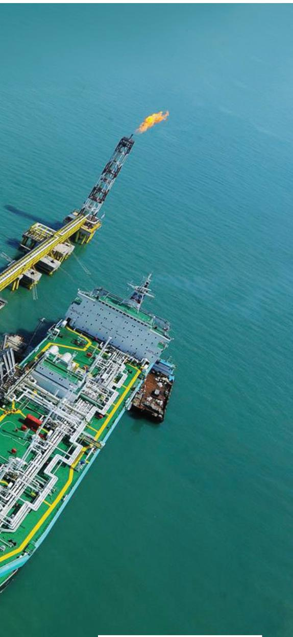
The world's first floating Liquid Natural Gas (LNG) regasification terminal (RGT) located in Sungai Udang, Melaka was completed in 2013, and helped increase the availability of natural gas in the country. A second RGT is currently being constructed in Pengarang and is expected to enter full operation in 2017.
