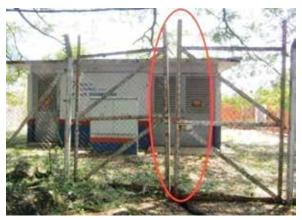
Substation gate is not closed securely
