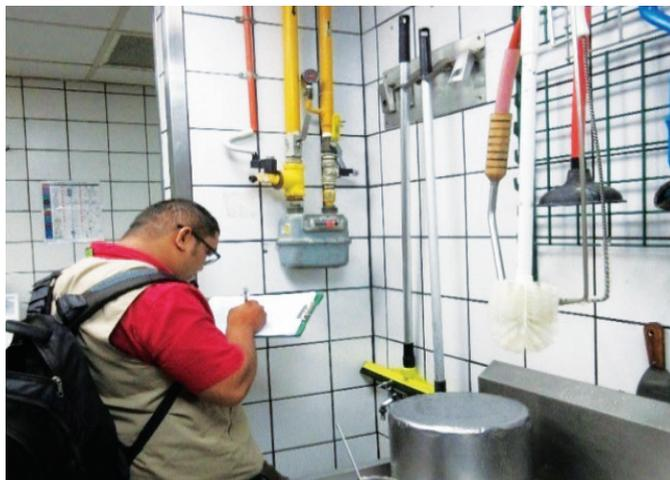
Checking a gas installation for proper maintenance and safe operation.
