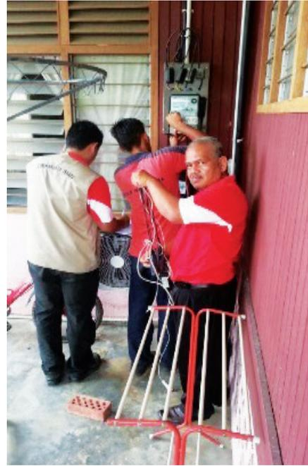
Checking on the accuracy of a meter at a premises suspected of having an illegal electrical extension.
