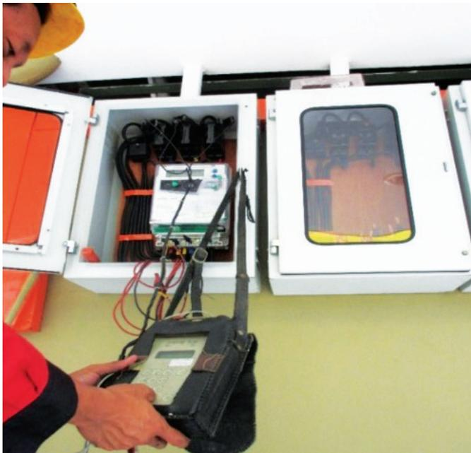
The Portable Working Standard equipment used to check the accuracy of electricity meters.
