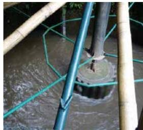
*The construction of a vortex system to generate power was supported by graduate students from University of Cologne in Germany. Besides generating electricity, the system can use excess electricity generated to pump water up to a series of 17 holding tanks at the top of the hill. The tanks can then be uncorked to flow water down the hill to generate electricity.*
