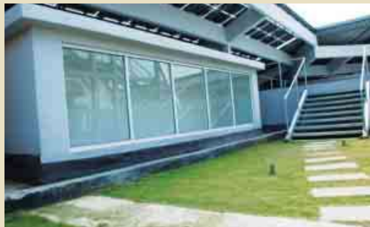
Roof light trough.
