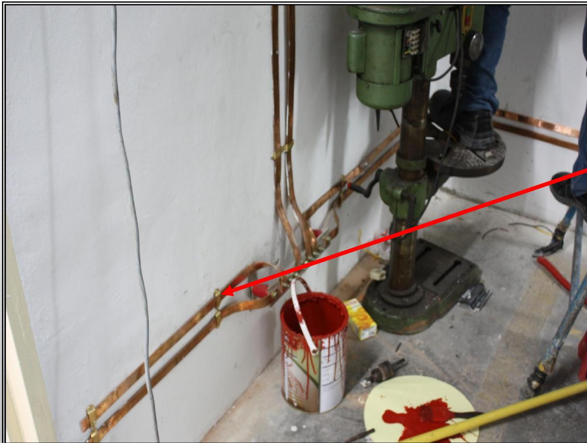
Installation of earth bar size 6mm x 25mm around the Tx room at 300mm from floor level.
