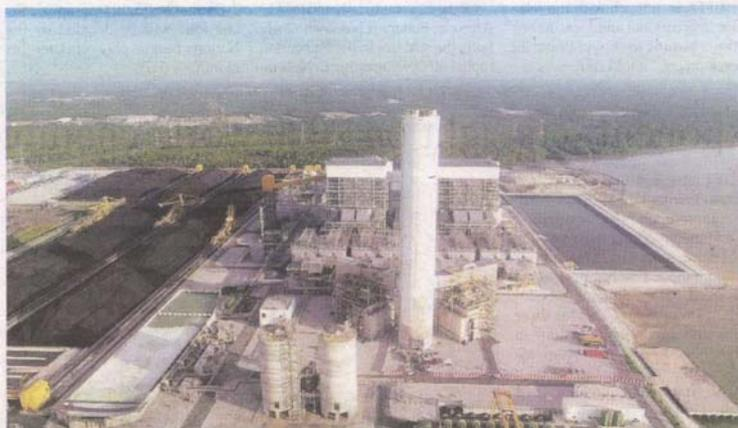
TMPS uses USC technology and is capable of producing 2,000MW at its peak performance
