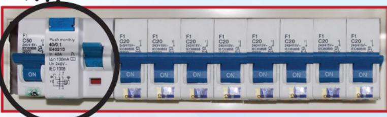
*Residual Current Device (RCD) is a protection device that protects consumers from electric shock and should be tested **AT LEAST ONCE A MONTH** to ensure that it works to cut off the circuit in the event of current leakages.*
