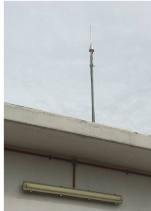
Building: Kuantan Medical Centre (KMC).
