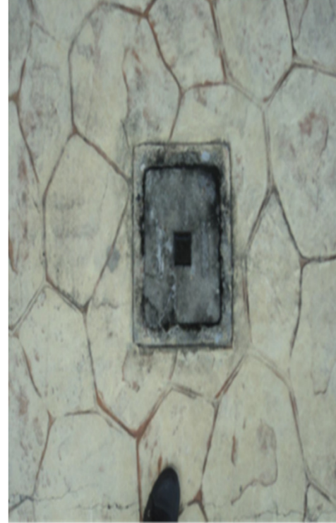
Building: DEMC Selangor Specialist Hospital.
